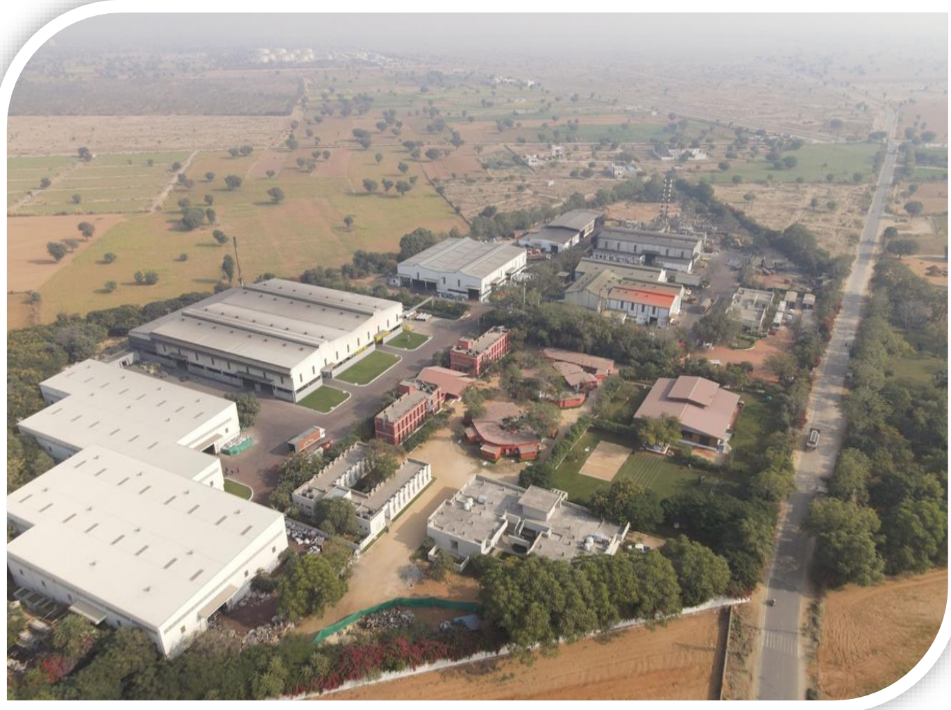
Phagi Plant's Full Ariel View
