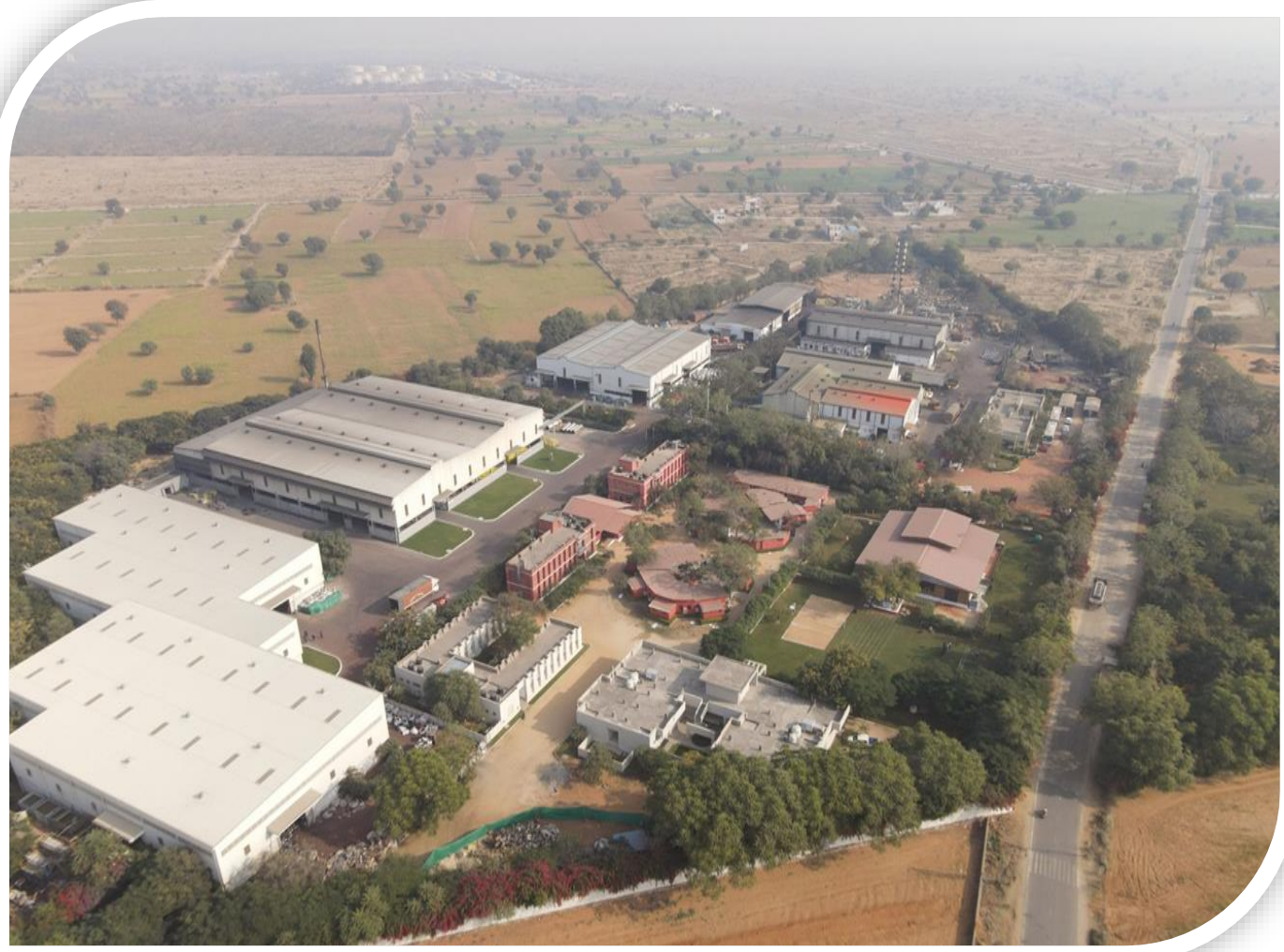
Phagi Plant's Full Ariel View
